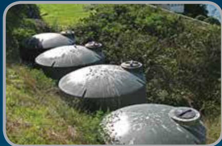
Parks use low-flow faucets and dual-flush toilets to conserve water. Parks use catchment tanks, like those pictured here, to collect and reuse rainwater. What can you do to help protect this precious resource?
