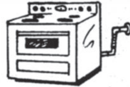
20. gas stove with rigid feed line
